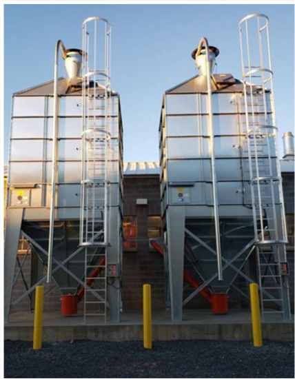
This Centralized Biomass Pellet Silo in Umatilla, Oregon, is an Oregon Army National Guard renewable energy project with a resiliency component which uses biomass from local forests for heating several buildings.
